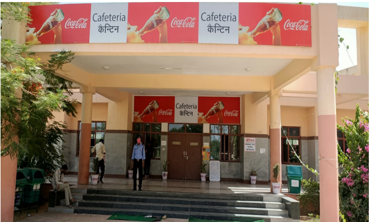
Cafeteria near IPD
